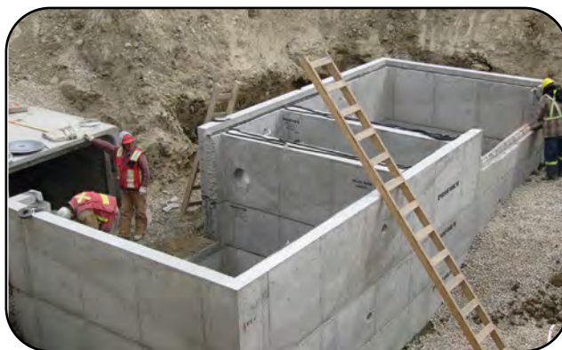
Our largest Precast Structure to date 29 x 10 inside to accomodate 2 - 10 x 8 Box Culverts c/w 2 weir walls.
