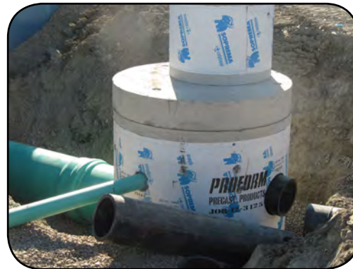
Can accommodate a variety of types of pipe with gasket connectors
