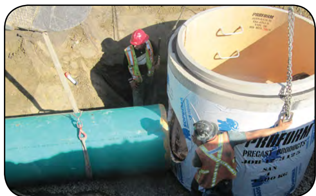
Insulated, Lined Manholes c/w A-Lok.
