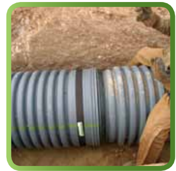
Bell/Spigot Joint Connection
