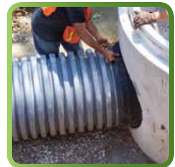
Manhole Boot Connection with Corrugated Pipe Adapter
